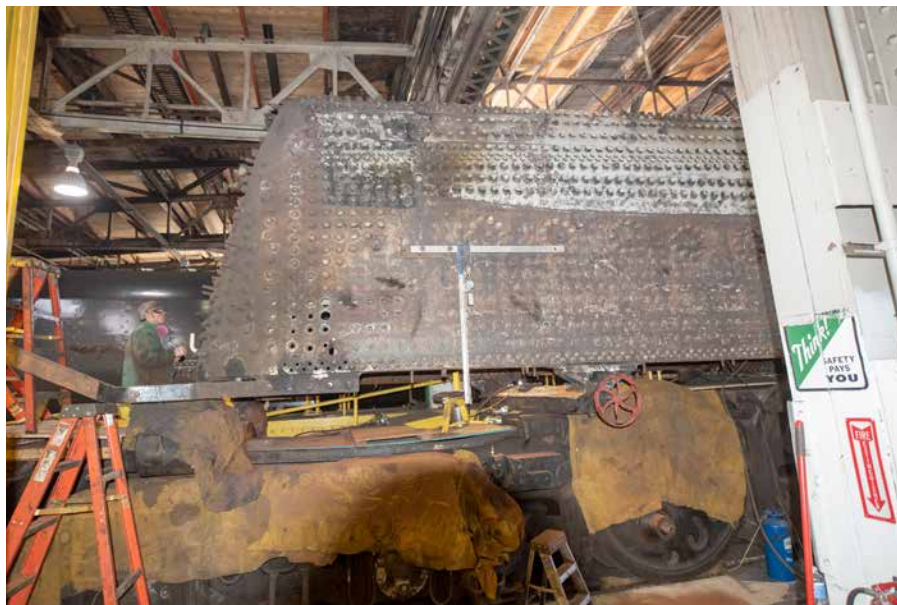
With the cab removed and the backhead exposed, work progresses on No. 4014's boiler in March 2017. Compare this image to the photos on page 149 showing the cab being installed in this area. Four photos, Jim Wrinn
