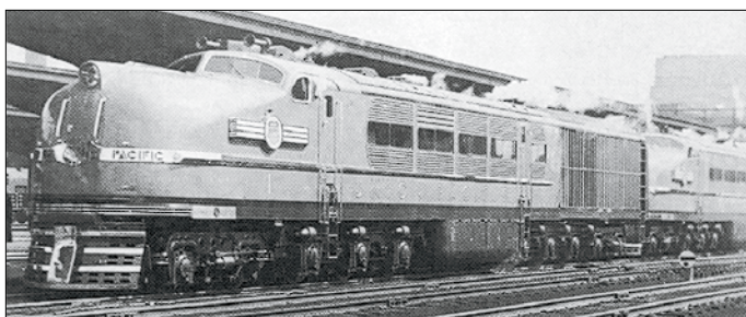
Steam turbine — Union Pacific 1 and 2 await departure from Omaha on their first run in March 1938. John P. McGlynn
