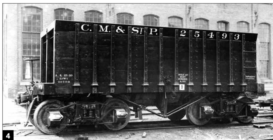
4 Chicago, Milwaukee & St. Paul 25493 was built at the railroad's West Milwaukee shops in 1900. The 50-ton car has wood sides, steel posts and underframe, and archbar trucks. Milwaukee Road
