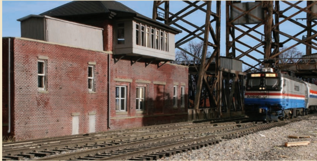
A northbound Amtrak train approaches the tower on the north shore of the Passaic River in Newark, N.J. In this case the brick on the tower was created using a dry-brush technique. A few individual bricks have been painted here and there for variety and contrast.
