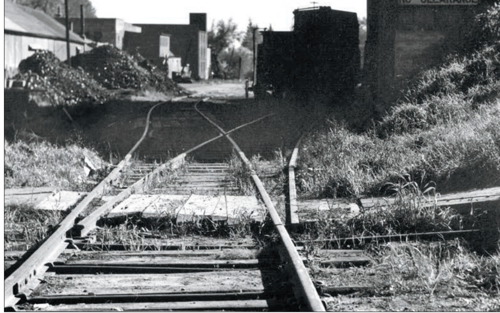
On a stub switch, the switch stand moves the approach rails, aligning them end-to-end with a route (the track to the left in this case). A misaligned rail is a serious problem. Paul H. Schmidt
