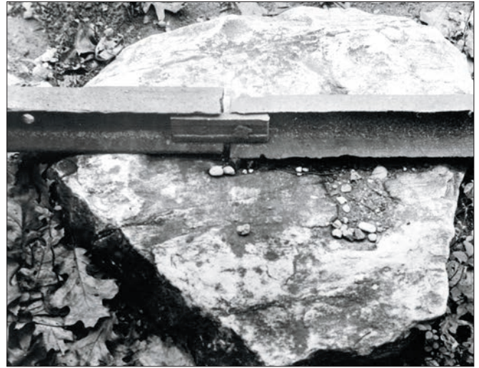
Early rail was often secured to stones instead of wooden ties. This is from a stretch of Camden & South Amboy dating to the 1830s, with 40-pound T-rail (rolled in England). The C&SA became part of the Pennsylvania Railroad. Pennsylvania Railroad; courtesy Association of American Railroads
