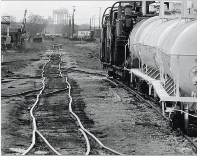
Not all track is well maintained. The jointed rail and turnouts in the Rock Island yard at Dallas, Texas, in 1977 is definitely slow-speed territory. Note the lack of ballast, as the track has sunk into the ground. Lee Langum
