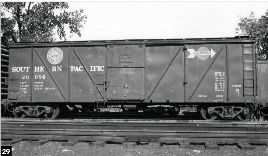
Southern Pacific's distinctive B-50-15 cars were rebuilt for Overnight service from older wood-sheathed cars with new steel sheathing. Note the ladder and stirrup at the door. Mainline Photos
