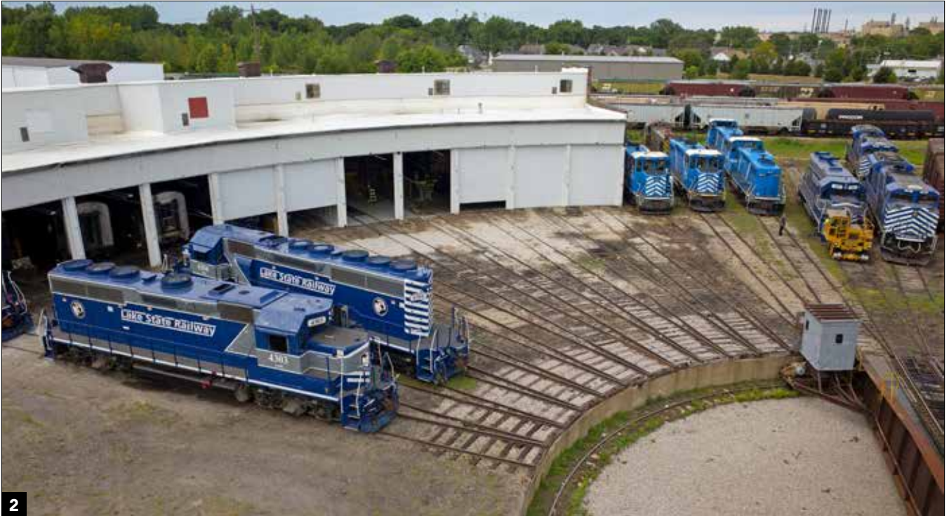
2 The Lake State Ry. uses the former C&O (Pere Marquette) roundhouse and turntable in Saginaw, Mich. It has replaced the classic swinging (and drafty) double doors with overhead garage-type doors. The Y-shaped 300-mile railroad operates between Flint, Saginaw, Bay City, Midland, Alpena, and Gaylord using a roster of second-generation EMD four- and six-axle power as well as new gensets. Chris Guss
