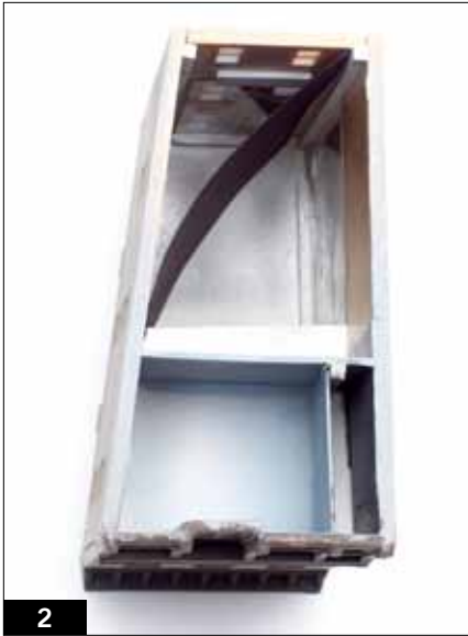
2 This building has both interior styrene walls and a construction-paper view block.
