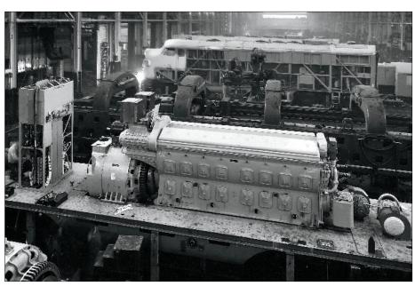
This 1949 view of the erecting floor at EMD shows a 567 diesel engine, generator (on the deck at the left end of the engine), and electrical cabinet (far left) in place on an F7 frame. An FP7 is taking shape in the background. EMD
