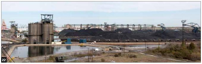
An overview of the coal loops at Newport News. The surge silos at the water's edge hold the coal being transferred to the ships.
