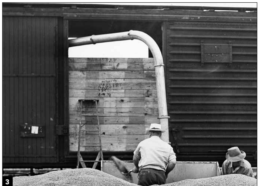
3 Workers load a boxcar with a conveyor in the 1940s. The wood grain doors are stenciled RETURN TO AT&SF. Jeff Wilson collection
