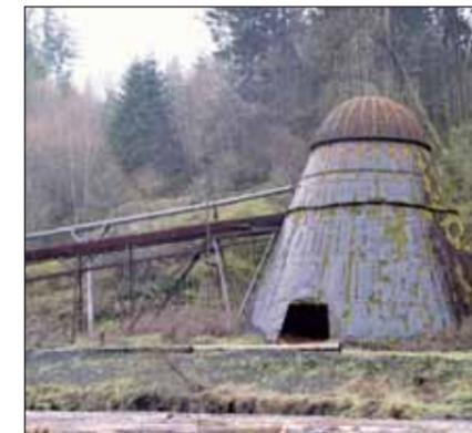
The Hull-Oakes "wigwam" sawdust burner could be found at most Western sawmills through the mid-1900s. The conveyor carried sawdust to the burner from the vacuum blowers at the head rig. Steve Austin
