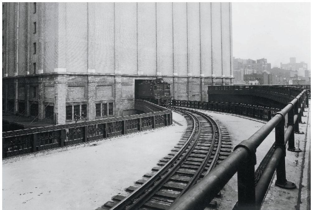
A tri-power locomotive switches at Merchants Refrigerating Co. at the south end of 10th Avenue. Elevated trackage included many similarly elevated industry spurs like those seen here. New York Central
