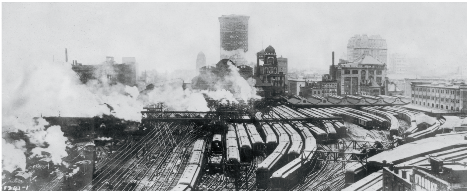
Smoke of 700 trains a day (date of this photo: Nov. 19, 1906) and a tunnel accident lead to electrification after the prohibition of steam in 1908. New York Central
