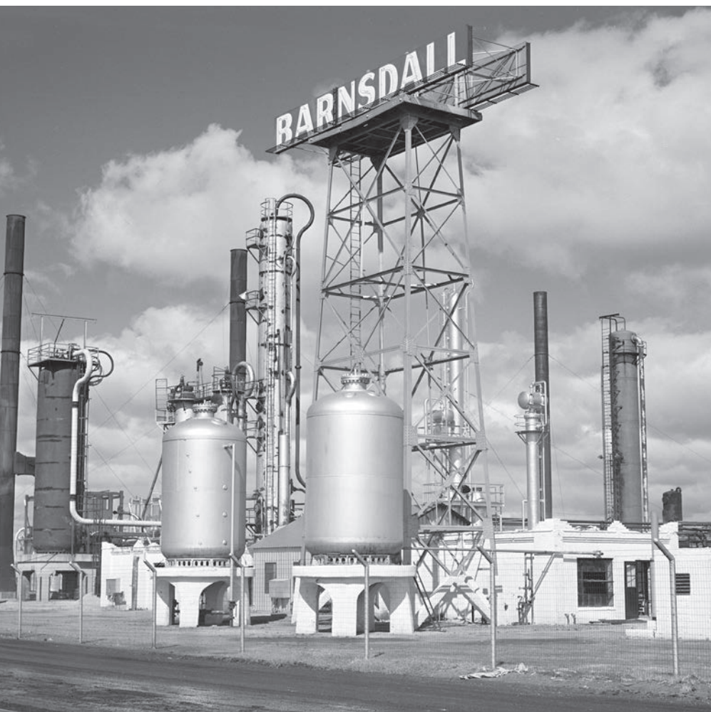
Typical of small refineries of the period, this Barnsdall refinery in Wichita, Kan., processed 5,000 barrels per day in the early 1940s. A fractionating tower stands just to the left of the tall sign. Marion Post Wolcott, Library of Congress
