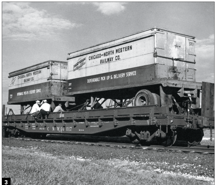
Workers tie down two short trailers on a 53-foot converted flatcar at the Chicago & North Western ramp in Green Bay, Wis., in 1954. Chicago & North Western
