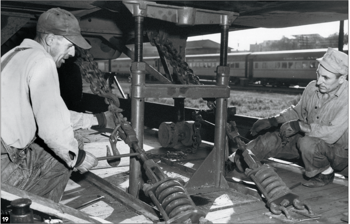
The pedestal jack has been positioned and raised under the trailer kingpin. The crew then attaches and tightens the chains. Chicago & North Western
