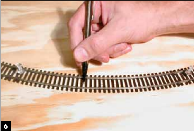
Mark the track center between ties every few inches (left). Then remove the track and connect the dots to mark the centerline.
