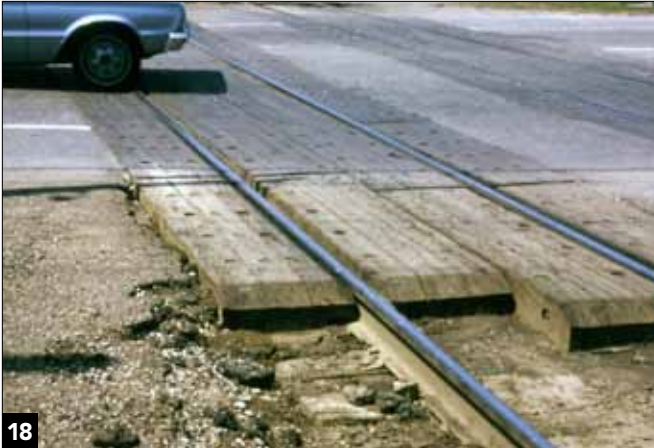
Highway crossings made from timber planks bolted to ties were the most common type through the 1960s. Gordon Odegard
