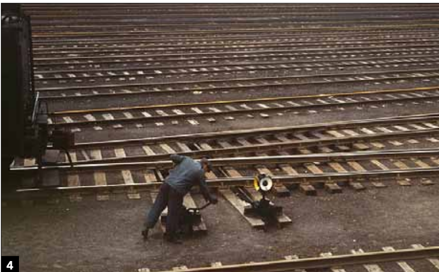
4 This 1940s photo shows a ground throw in the Chicago & North Western Proviso yard topped by a kerosene lantern. Library of Congress
