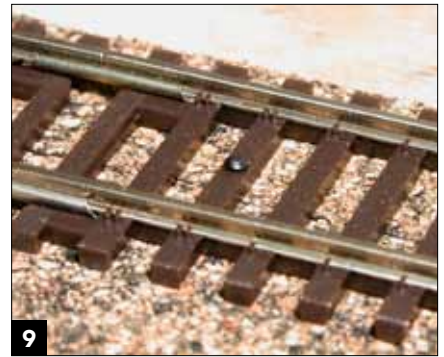
Leave a paper-thin gap between the nail head and the tie to avoid causing a kink in the tie.
