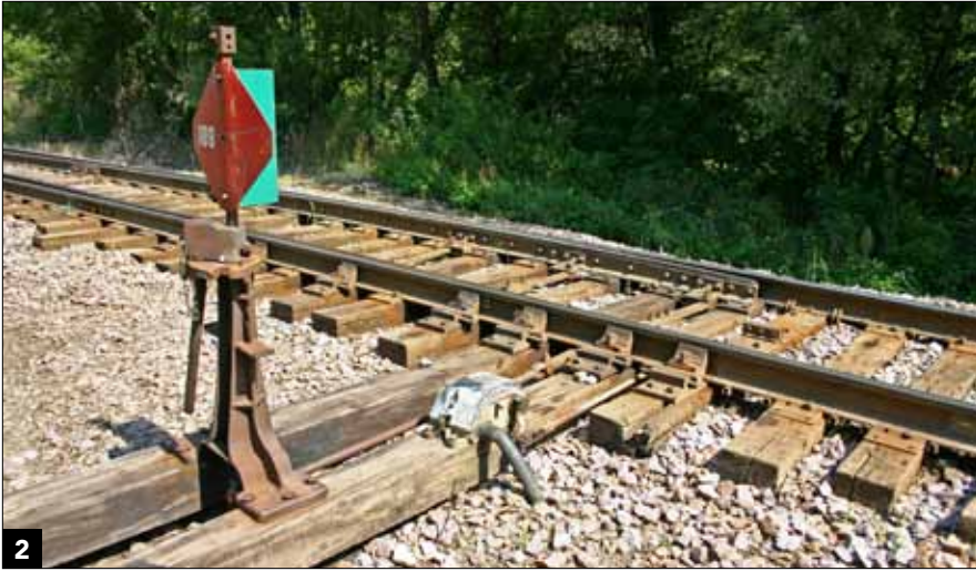
2 This modern intermediate switch stand on the Union Pacific leads from a main line to a grain elevator spur. A padlock protects the stand. The silver control box relays the switch indication to the signal system.
