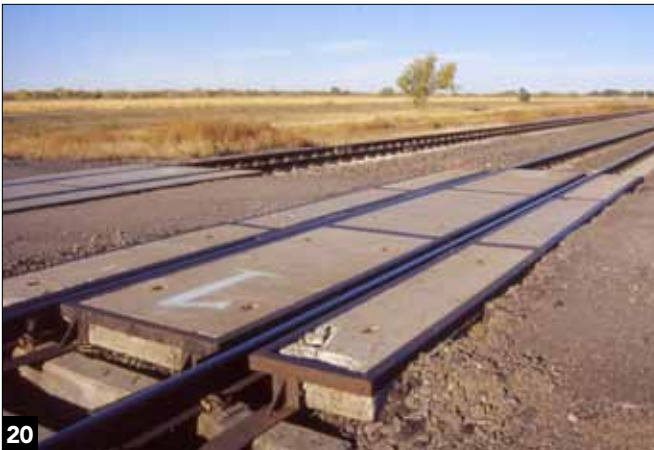
Crossings of concrete pads bolted to ties can be found in many modern installations.
