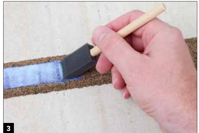
3 Mark the outside edges of the ties and spread a thin coat of white glue on the roadbed.
